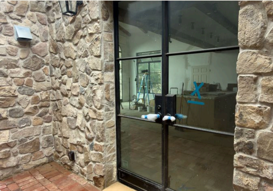
French door out of the kitchen
