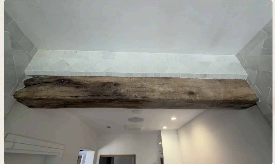
Beam we milled onsite from a coastal live oak that we lost in the fire, installed in the bathroom
