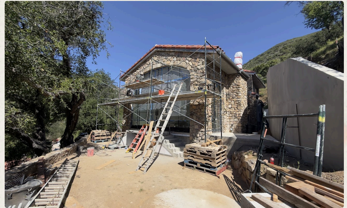
Stone veneer applied with mortar and anchors over MGO is the final exterior layer.
