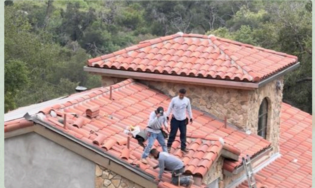
Mission clay roof tile being installed
