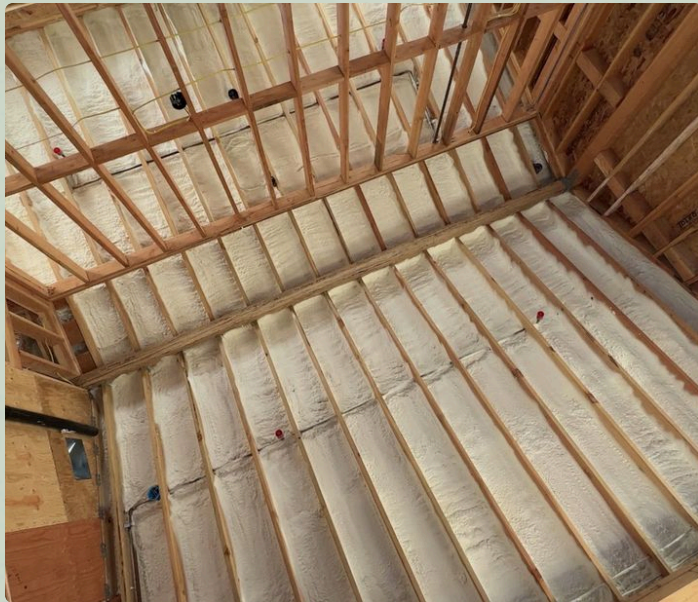
Ceiling: soy-based, low-Global Warming Potential (GWP) closed-cell spray foam (Huntsman Heatlok HFO EZ)
