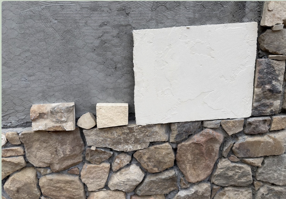
Testing limestone stucco samples with our salvaged stone veneer
