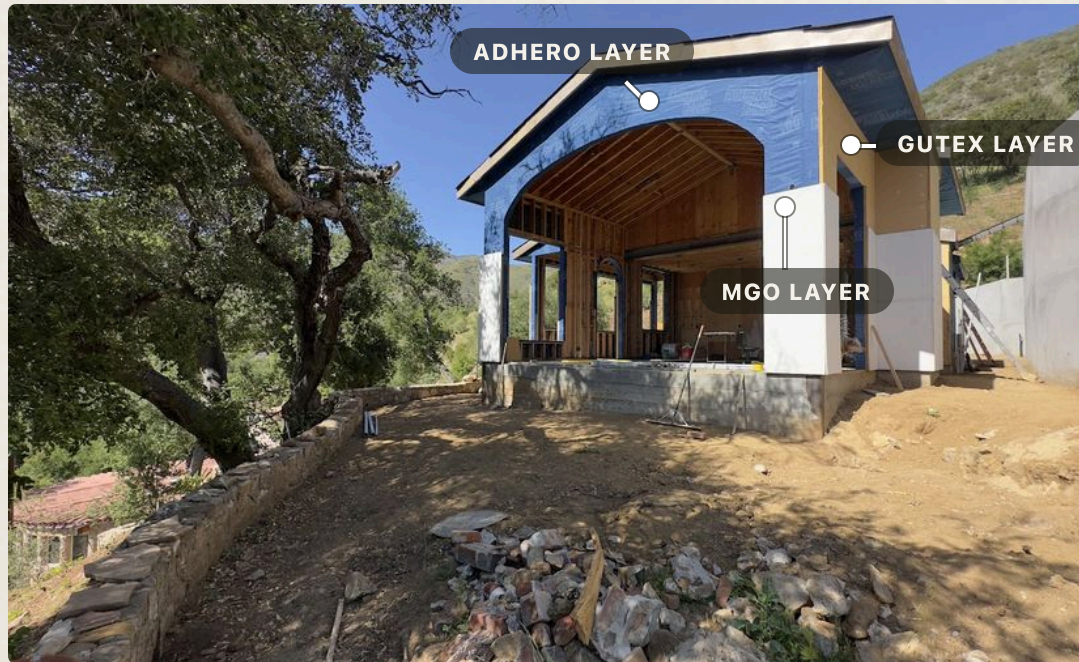
Living room window, with Adhero 3000 (over Gutex not visible in photo), then covered by MGO
