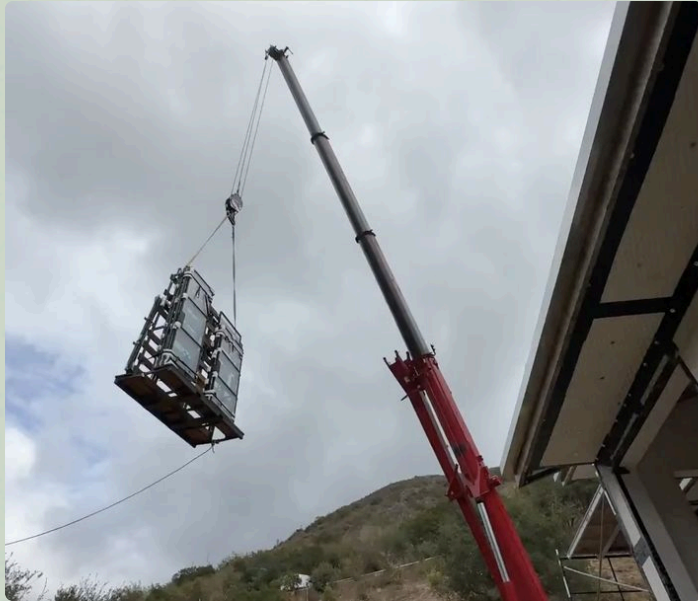
A finished window unit, craned into its opening
