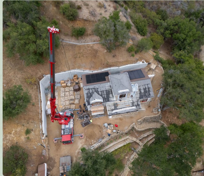
A crane was needed to lift the window over the house
