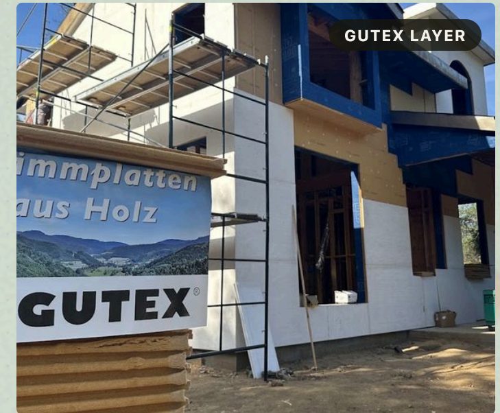
Walls: Gutex Multitherm 40mm / 1.57" wood-fiber board
