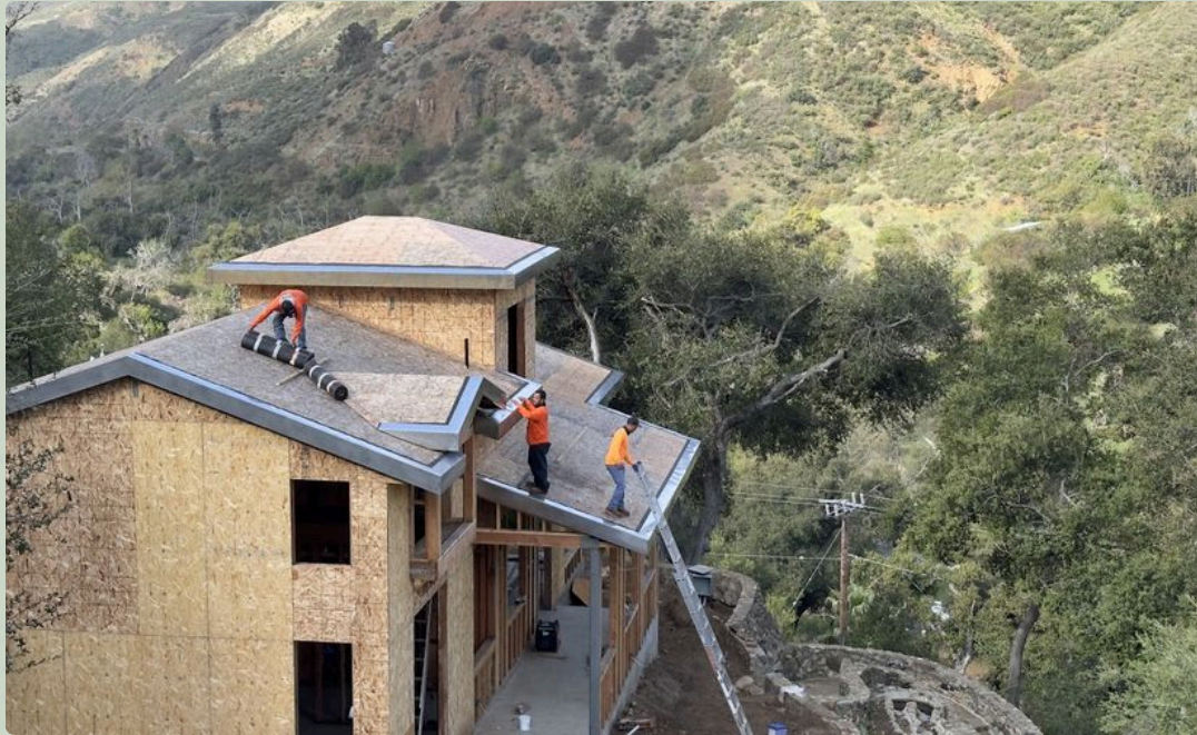
Polystick XFR WUI underlayment on the non-vented roof
