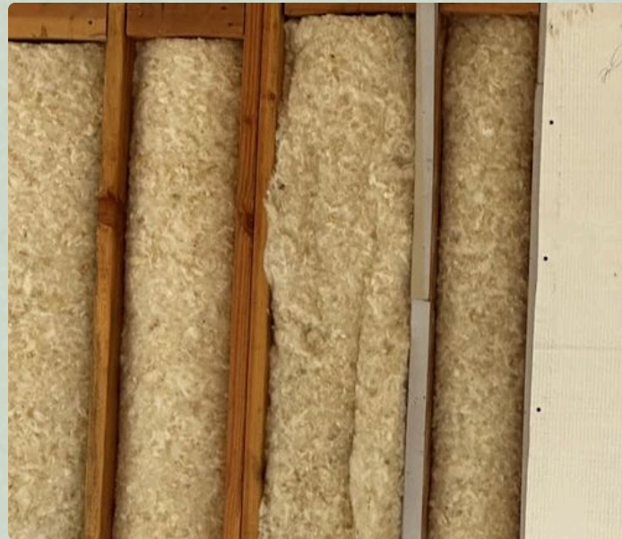
Ceiling & walls: Havelock R22 sheep wool batt
